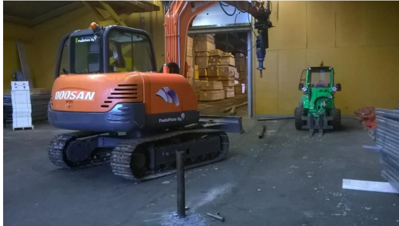
FOUNDATION- AND FLOOR STRENGTHENING
