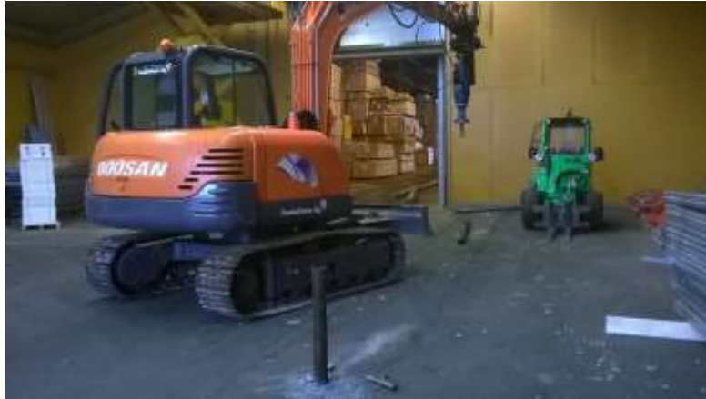
FOUNDATION- AND FLOOR STRENGTHENING
